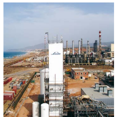
Helium recovery and liquefaction plant in Skikda, Algeria
