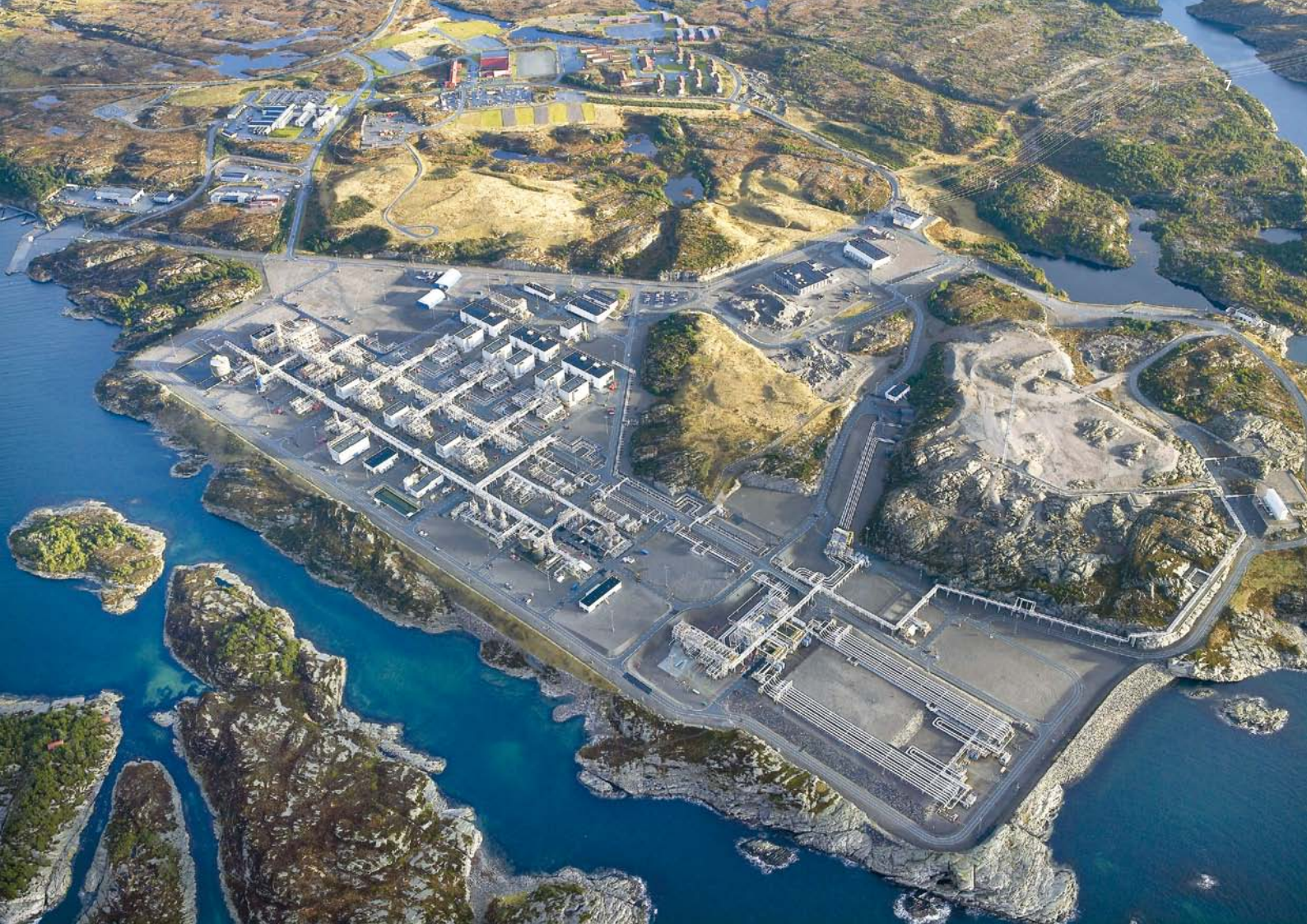
C 3+ recovery plant in Kollsnes, Norway (Photo courtesy of STATOIL)
