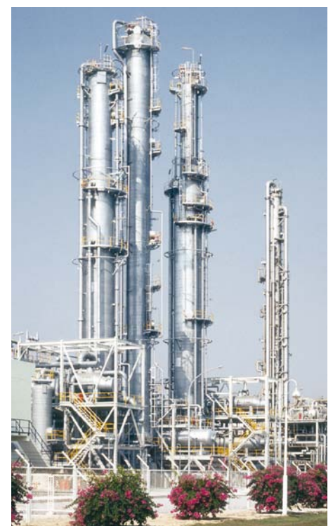
C 3+ recovery and fractionation plant in Rayong, Thailand
